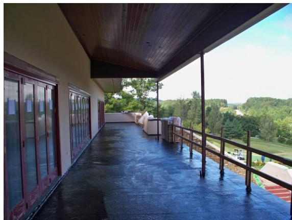
Waterproofing at balcony topping slab
