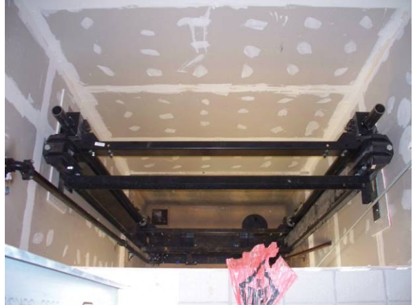
Freight elevator progress
