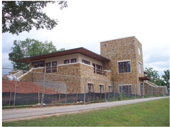
Progress from east golf course
