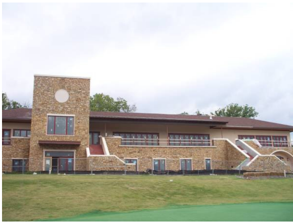
Progress view from putting green
