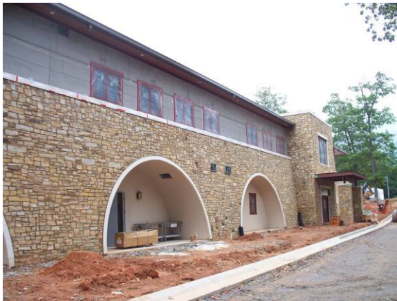
Main entrance progress view
