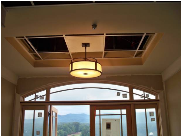
Light fixture entry
