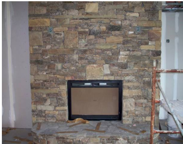
Fireplace at 2 nd floor community room
