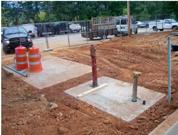
Water vault installation
