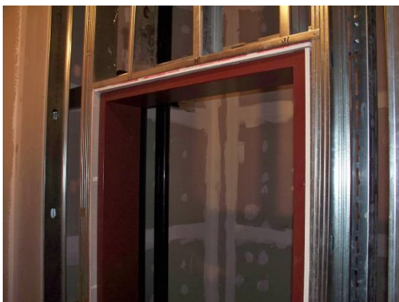
Door frame for passenger elevator at 1 st floor lobby
