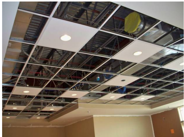
Ceiling grid and lighting
