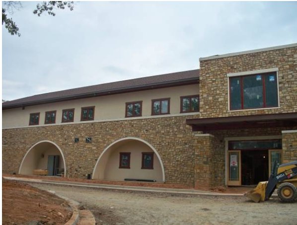
Main entrance progress view
