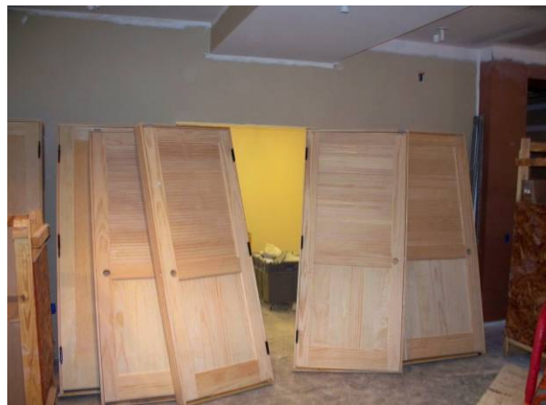
Wood doors ready for installation.
