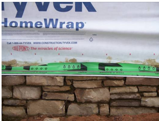
Exterior Waterproofing and Flashing
