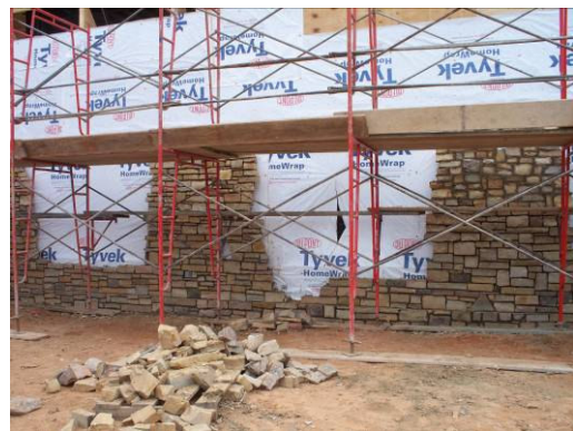
Exterior Stone Installation
