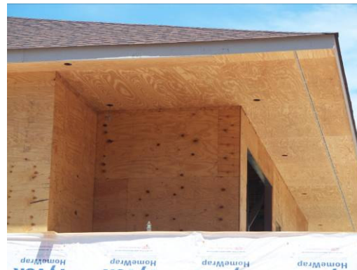
Exterior Sheathing and Eave Framing
