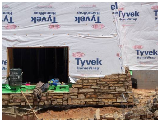
Exterior Stone Installation
